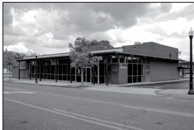
Post-war Modern style buildings are typically more streamlined in style, with minimal ornamentation, expanses of glass, and often overhanging flat roofs.
