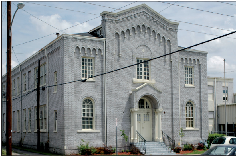
Ensley First Presbyterian Church Building 616 21st Street • Resource #60 • circa 1920 • now A.C.T.S. Ministries, Inc.
