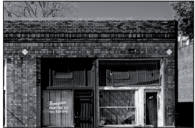
Early 20th Century commercial buildings often feature patterned brickwork with little or no relief, decorative inserts, and the use of prism glass in transoms.
